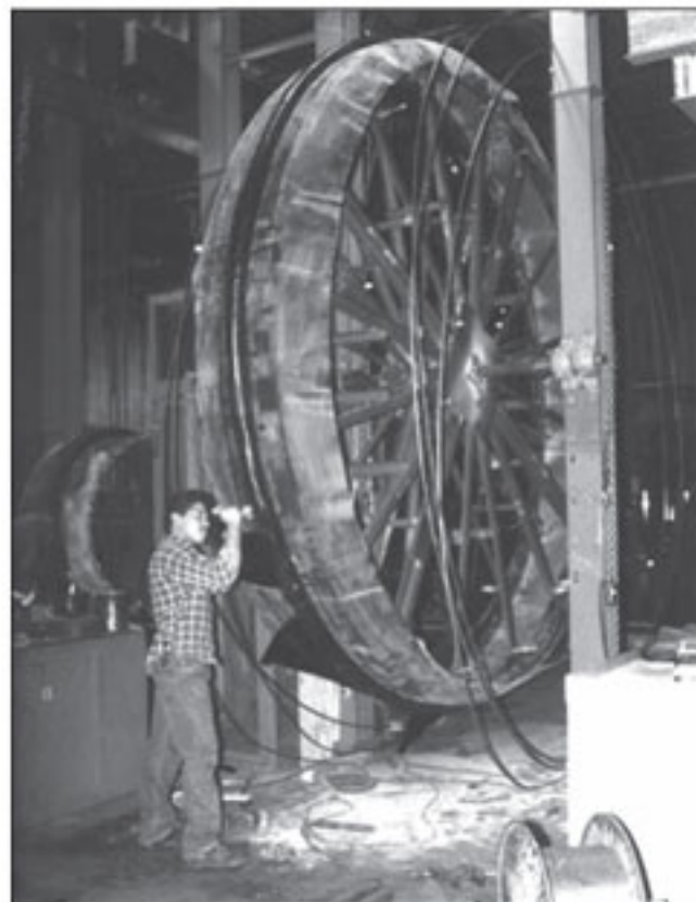
A huge 132" (3353mm) diameter single arch 501 under construction. Very few manufacturers have the equipment or the engineering staff to work to these diameters.
