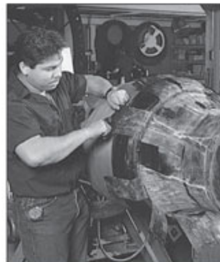
Pulling the tire cord reinforcement from one steel arch reinforcing ring, across the arch to the other ring adds to arch strength and shape stability.
