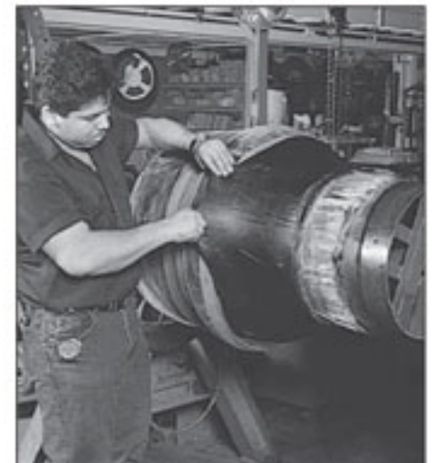
Pulling back cover, tire cord reinforcement and tube prior to building the flanges on an eccentric reducer.
