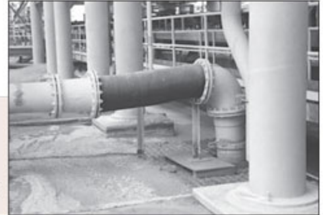
Series 100 flexible hose installed in a cooling tower return line. Notice the major vertical displacement to compensate for the misaligned piping.
