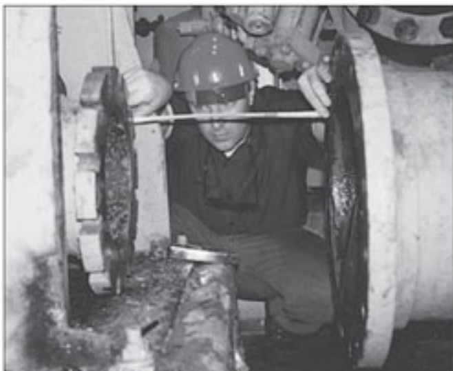
Measurements being taken for a retrofit. The eccentric reducer was manufactured to the exact length with non-parallel flanges. The photo at right shows the reducer after installation.
